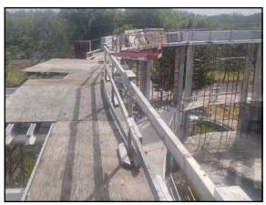
to Column; and then we will install the 30" wooden Wall Forms on both sides of the Beam Rods.
